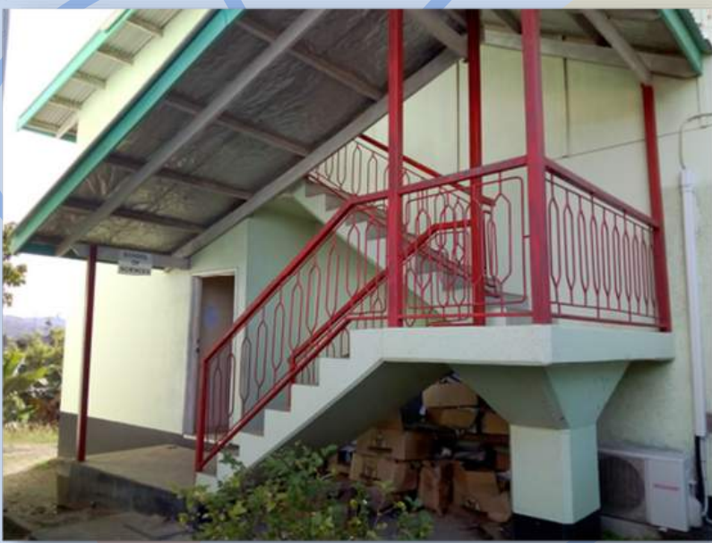
The School of Sciences (SOS) main office building located at the Panatina Campus, East Honiara.
